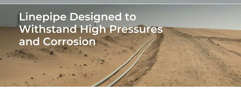
Constructed from a winning combination of high-density polyethylene, helically wound epoxy-free dry fiberglass and a protective outer jacket, Flexpipe products are safe to install thanks to smaller crew sizes and less heavy equipment requirements.
